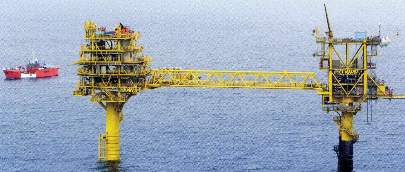
The Valdemar Field after installation of the Valdemar AB platform (left) and the bridge connection to the existing platform.
