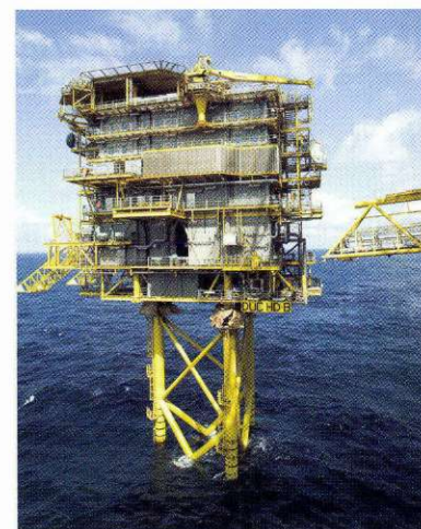
The new accommodation platform has been installed on the Halfdan A Field, and the bridge to the processing and wellhead platform is being lifted into place.
