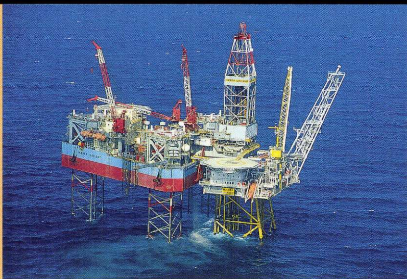
With a leg length of 183 metres the MÆRSK GALLANT can operate at water depths up to 125 metres in the harsh environment of the North Sea. The "excess" leg length is necessary to keep the hull out of reach of the waves.
