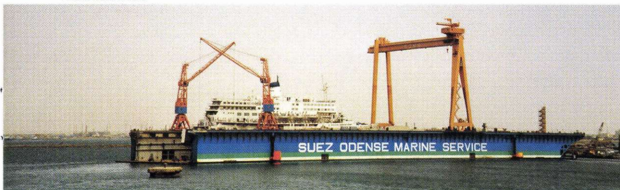
On the west bank of the canal Suez Odense Marine Services' impressive floating dock is situated, owned by the Odense Steel Shipyard together with the Suez Canal Authority. The floating dock, which has a lifting capacity of 55,000 tons, is one of the world's largest. It is described in more detail in Mærsk Post 4/97.
