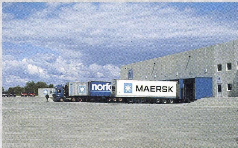
The new terminal in the Port of Copenhagen handles all forms of cargo for transportation in containers, trucks, swap bodies and trailers.
