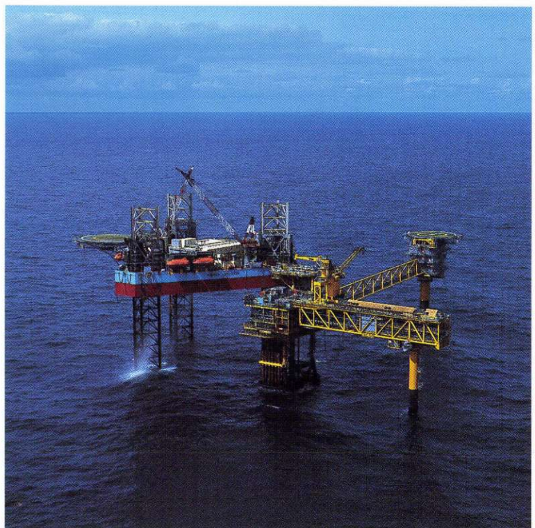
The Skjold Field after completion of the expansion programme in June 1994. On the right is the accommodation platform, MÆRSK EXPLORER which, during the busy development period, accommodated the many persons involved in the project.
