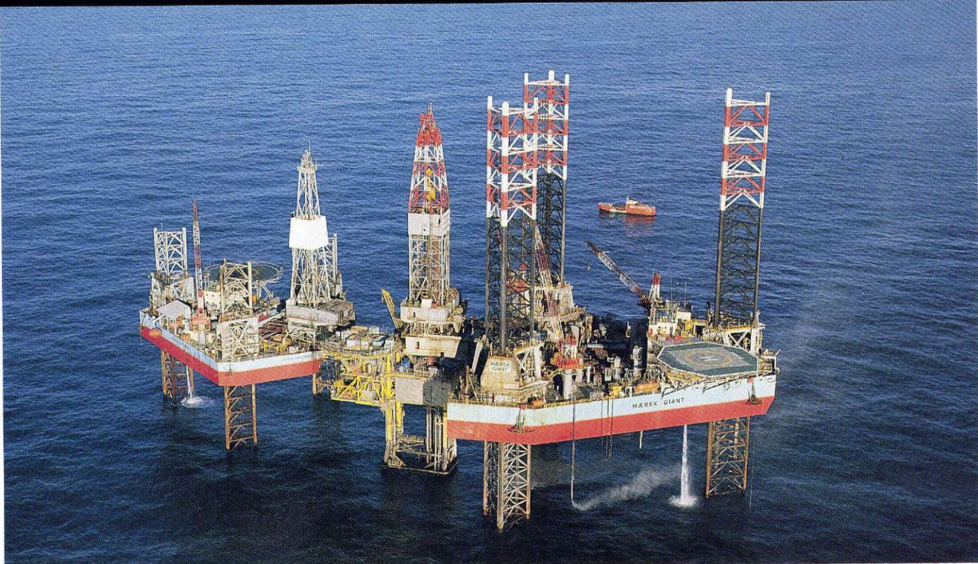
The drilling rig "MÆRSK GIANT" – one of the largest jack-up rigs in the world – takes up a great deal of space in the Skjold field, where its derrick towers over the production platform. On the left is the somewhat smaller drilling rig "MÆRSK EXPLORER", which supplies purified sea water for injection in the Skjold and Gorm fields.
