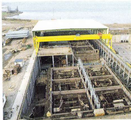
Dock 3 with the newly-installed cover, which provides shelter from wind, rain and snow. The platform in the middle is the place of delivery and the gantry crane is used both to lift the hatch covers and to transport the working materials.
