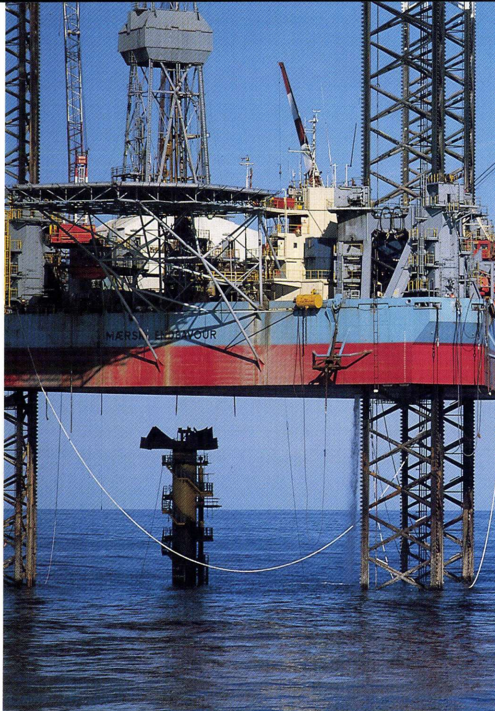
The most critical part of the operation has been completed – the platform is now standing on the sea bed, and the next phase of the installation can soon begin.
