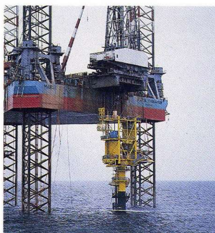
The installation has been successfully completed and the last stage of the operation is to lift the top module into place.
