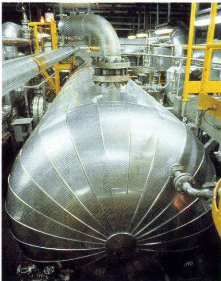
Salamis insulation work on a offshore platform.
