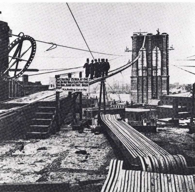
Trustees of the Brooklyn Bridge Company on the Brooklyn end of the footbridge used for stringing cables.
