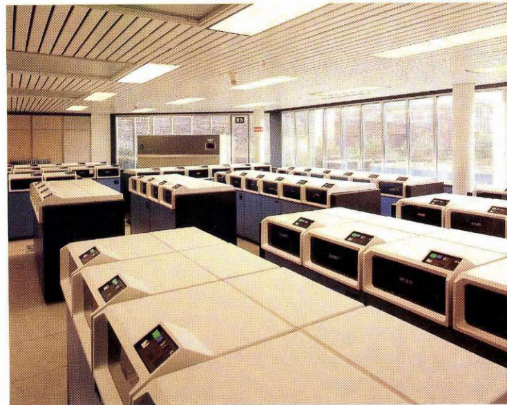
A section of Mærsk Data's about 90 disc drives – direct access storage devices – able to store almost 30 billion characters.
