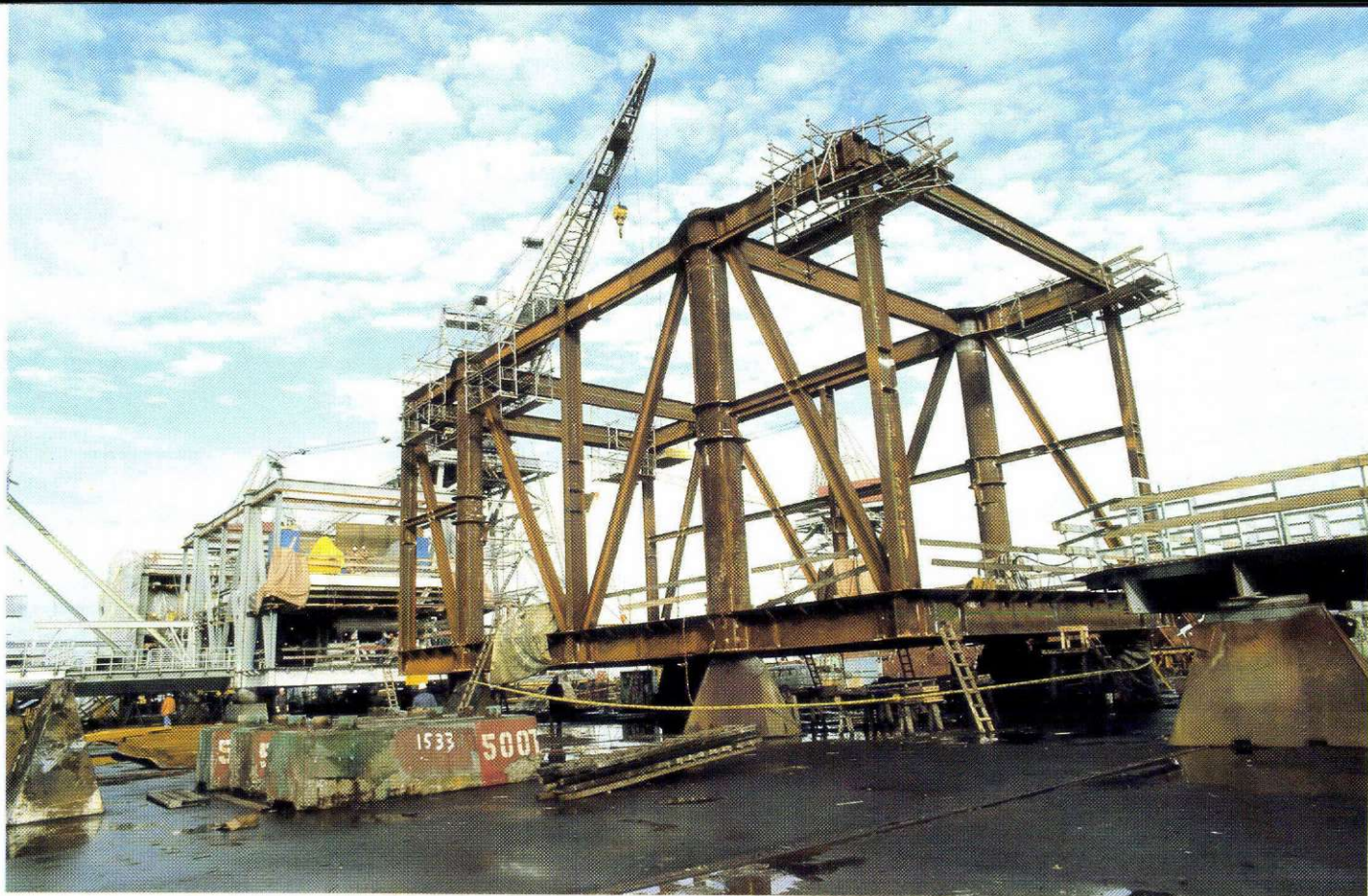
Three of the eight Lindø modules for Tyra East at various stages of completion.
