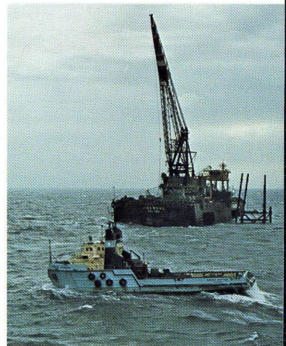
The gigantic floating crane "NARWHAL" operating in the North Sea. On the right is the top of a platform section positioned on the sea-bed by the crane.
