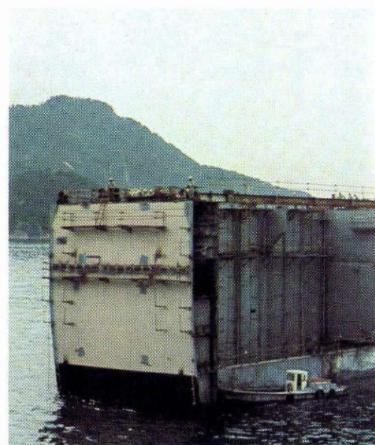
The forepart waiting outside for the new mid section to be towed in.
