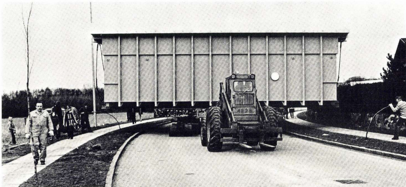
The Lindø Yard's transport section is used to negotiating nooks and corners. But they needed all their skill for the transportation of the pools from the Yard to the building-site at Munkebo. Young trees were bent to give passage.
